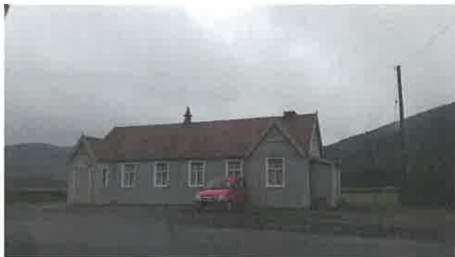
Ettrick Village Hall
